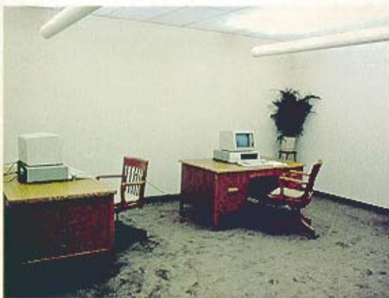
The same room lit with a Peerless system. The even wall and ceiling illumination takes the hot spots off the screens.
