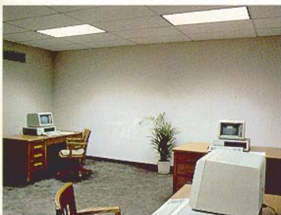
The University of Colorado test room lit with parabolic fixtures. Note the glare on the screen of the VDT on the right.
